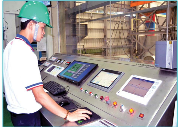
Control Room of Extra-High Voltage Test Laboratory
